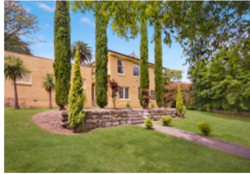
7 Hinkler Street, Greenwich
